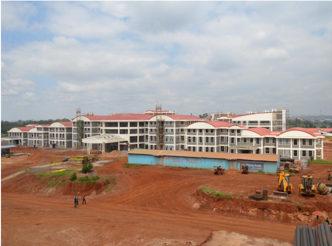
Ongoing construction of the referral hospital
