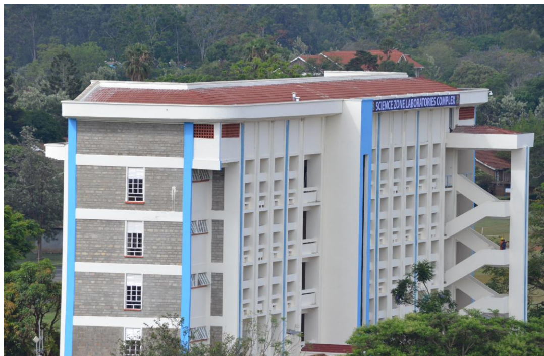
Science Zone Laboratories complex
