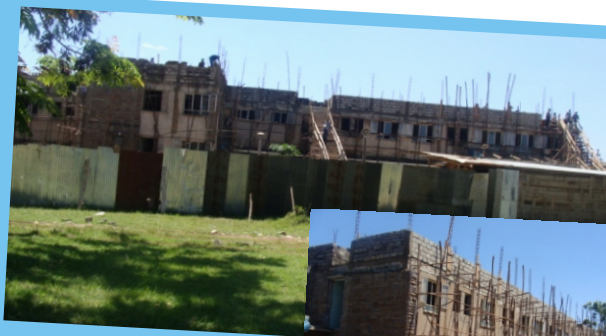
The on-going rehabilitation of the double roomed, self-contained Suswa Hostels.
