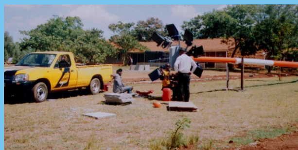
Adopt-a-Light technical staff install another floodlight at the Nyandarua Hostels area.
