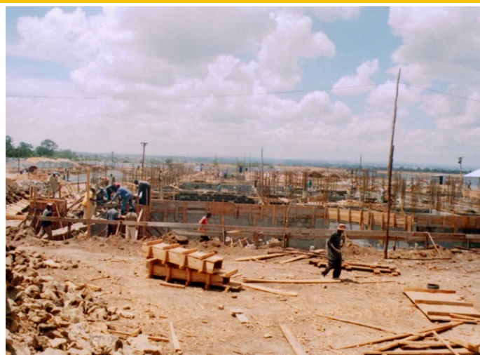
School of Engineering Construction site.
