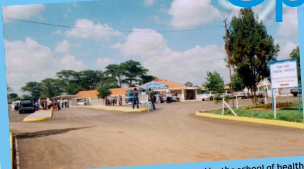
The new Thika Road Funeral Services managed by the school of health sciences now fully operational.
