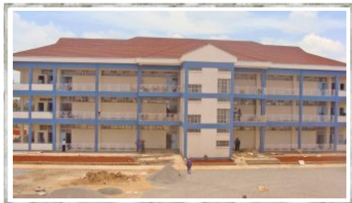
The three storey building which is constructed near the Science Complex (A.V.U) has six laboratories each with a capacity of a hundred students. It also houses technician's offices.
