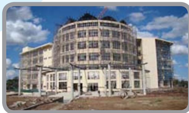
The new Library nearing completion.
