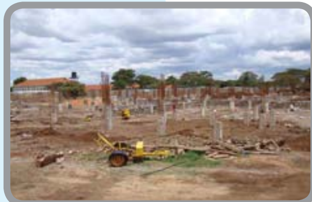
New Administration Block in progress.
